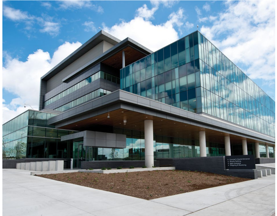
Forensics Services Coroner's Complex, Concert's first public-private partnership project, Toronto, Ontario.
