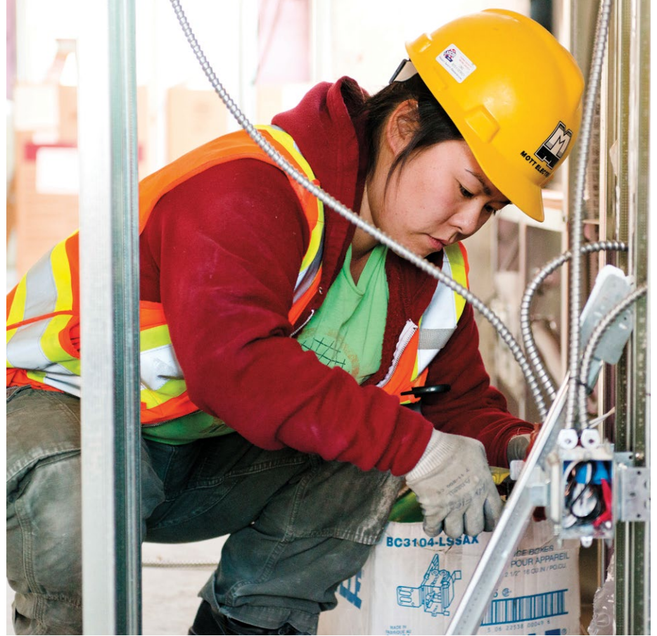
An electrician works on Salt, Vancouver.
