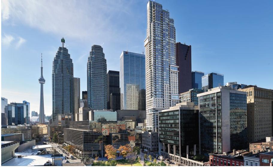
88 Scott, a mixed use 50 story tower targeting “Tier 2” of the Toronto Green Standard.
